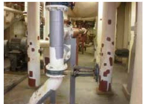
Spot repaired surface on pipeline
