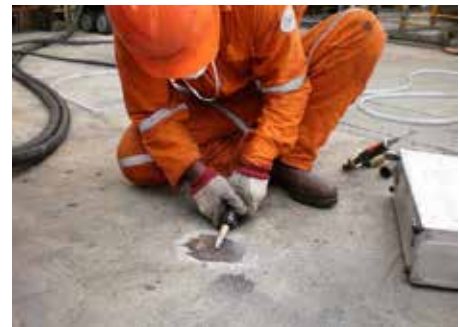
Spot repaired surface on deck
