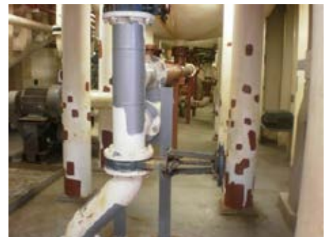
Spot repaired surface on pipeline
