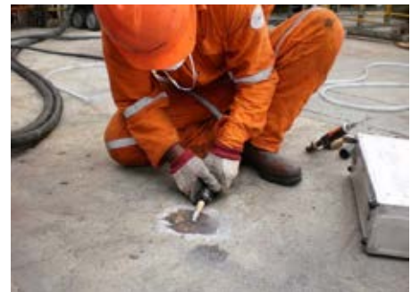
Spot repaired surface on deck
