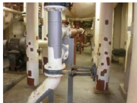
Spot repaired surface on pipeline
